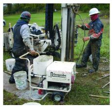
Technicians working for Textron use a "direct push" Geoprobe® grout machine to seal a borehole that was used to evaluate the subsurface groundwater near the Acument Global Technologies plant in Rochester, IN, a plant formerly owned by Textron. A work plan Textron submitted to state environmental authorities calls for a network of permanent groundwater monitoring wells at 27 nearby locations.
